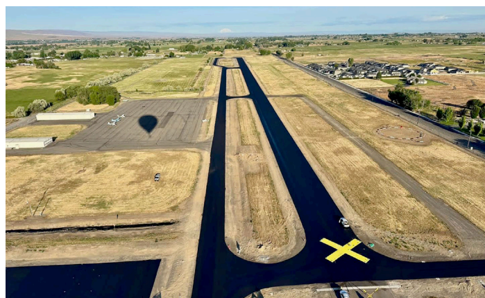
Prosser Airport Lighting & Replacement Project
