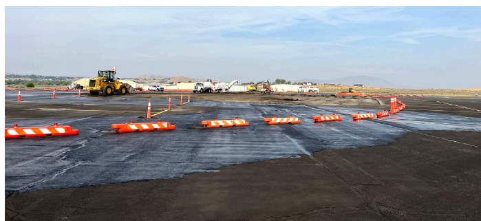
Richland Airport Apron Improvement Project
