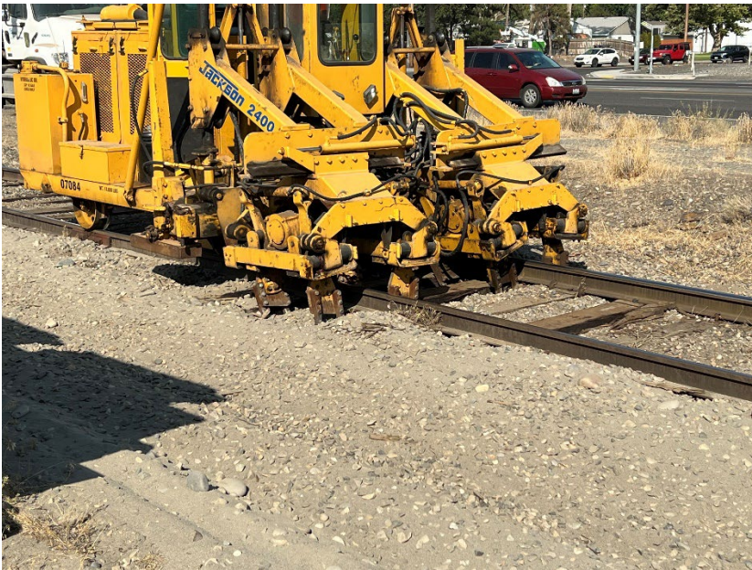
Tamping new ballast
