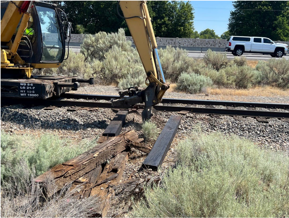
Tie Inserter installing new ties
