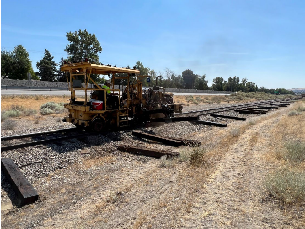
Tie inserter installing new ties
