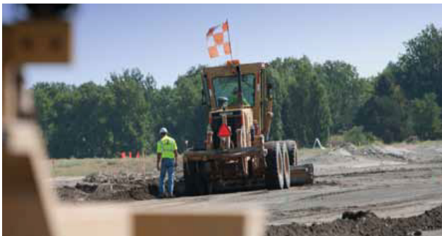
Contractors prepare the ground to relocate taxiway B at the Richland Airport.
