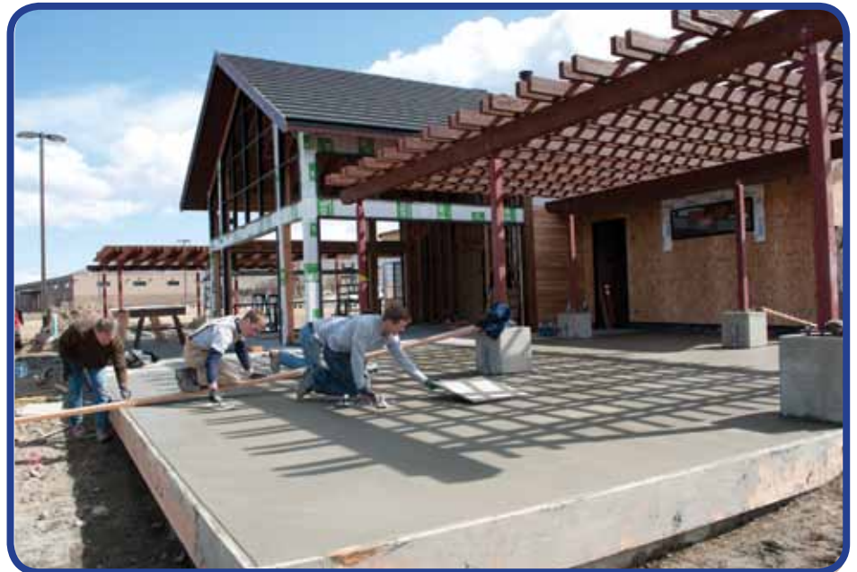
Above construction shows George Booth & Sons Construction workers smoothing the patio.
