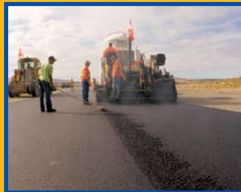
The main Richland Airport runway (fondly referred to as the roughest run in the west) is being reconstructed. Inland Asphalt, a local Richland company, was hired to complete the task, which includes removing 47,500 square yards of old asphalt, placing storm drain pipes, building dry wells, removing and reconnecting runway lights and signs, modifying taxiways and laying 30 tons of aggregate base and 20 tons of surface material.
