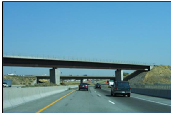
Berry's Overpass Bridge
