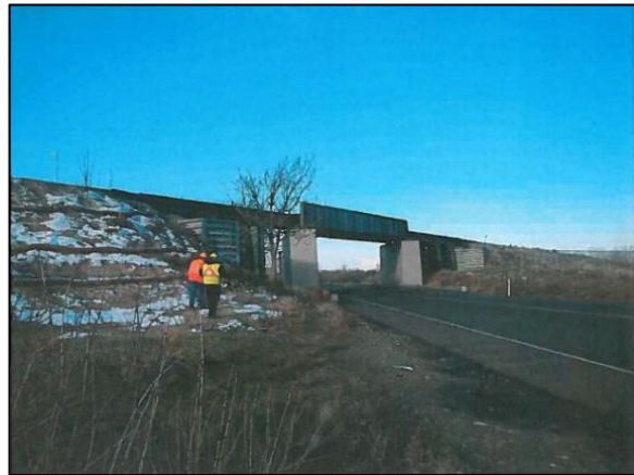
Columbia Park Trail Bridge
