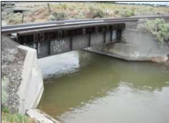
Irrigation Canal Bridge
