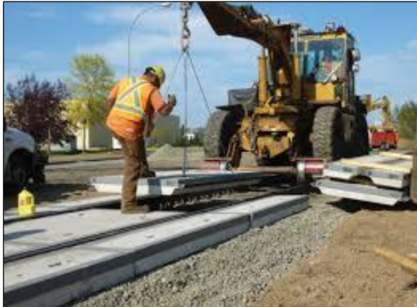
Speed Swing placing Concrete Panels
