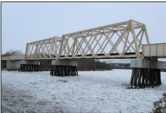
Yakima River Bridge
